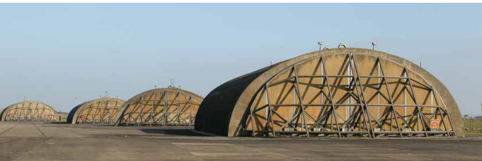
The hangars at Upper Heyford
